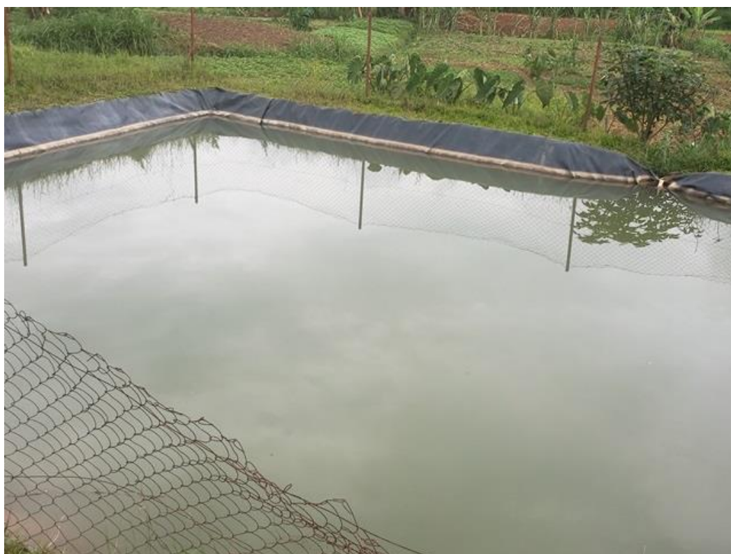
Figure 4: Typical Water ponds found in Rwanda (lined with plastic sheeting)
