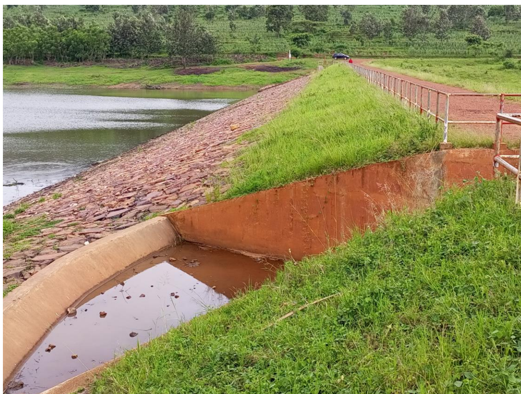
Figure 12: View of Rwinkwavu embankment dam
