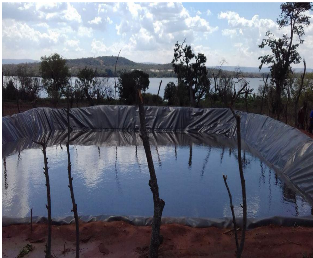
Figure 2: Water pond lined with plastic sheeting
