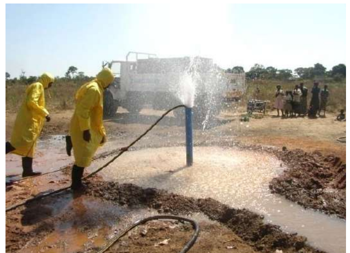
Figure 9: Cleaning the borehole with an air-jetting tool
