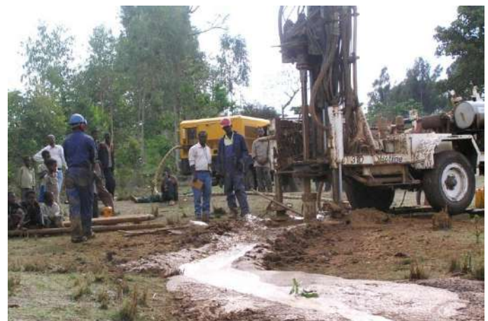
Figure 12: Drill rig with drilling fluid channel
