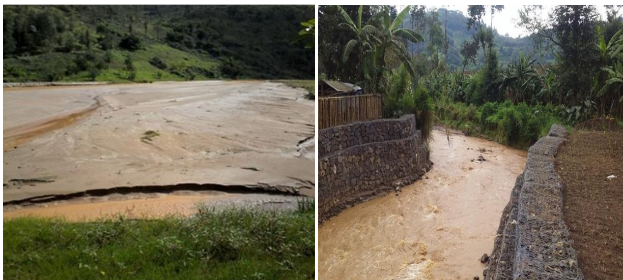
Picture 2: Erosion and sediment transport in Secoko River (left side picture) and in Sebeya River at Pfunda Tea factory (right side picture) for protecting the factory against stones and soil transport within Sebeya River which have been destroying and flooding the factory compound for years.
