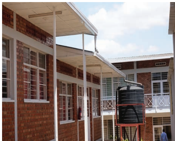
Plastic tank used for storage constructed above ground
