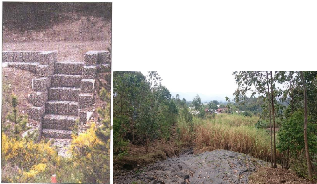
Figure 140: Gabion boxes weir (left) / Natural bedrock fall on Susa River (right)
