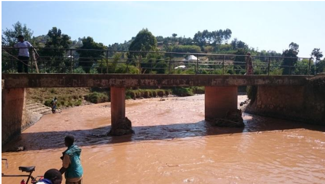
Figure 131: 15m span slab bridge on Sebeya river
