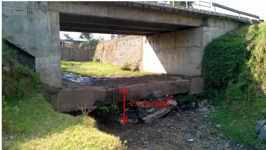
Figure 117 Rwebeya bridge in Musanze-city
