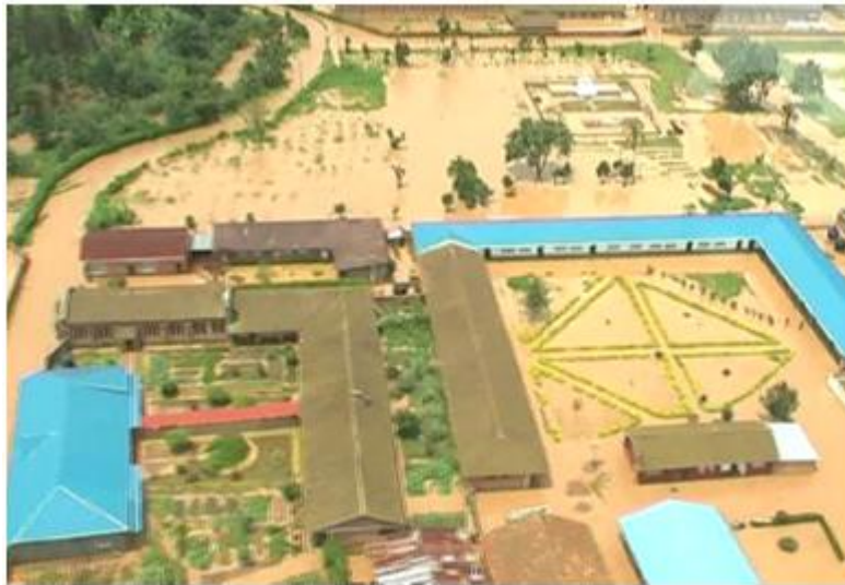
Figure 68: Flooding of the school "petit séminaire" 2 (no date)
