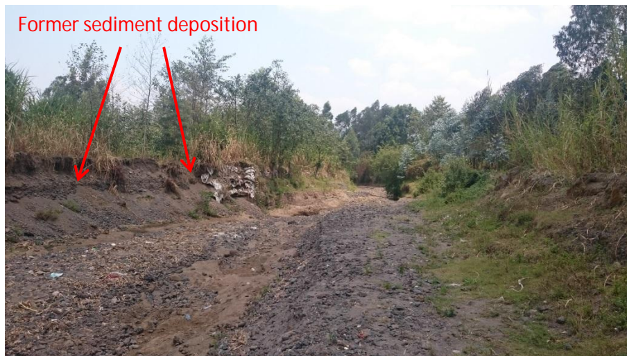
Figure 122 Area to be reworked into a debris basin (downstream view)
