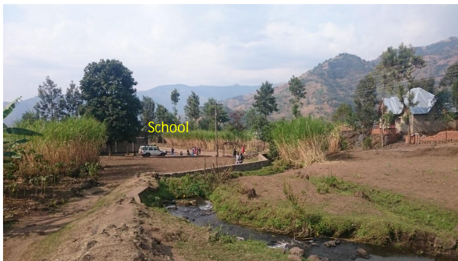
Figure 47: Mutobo left reach: dike overflowed in 2014
