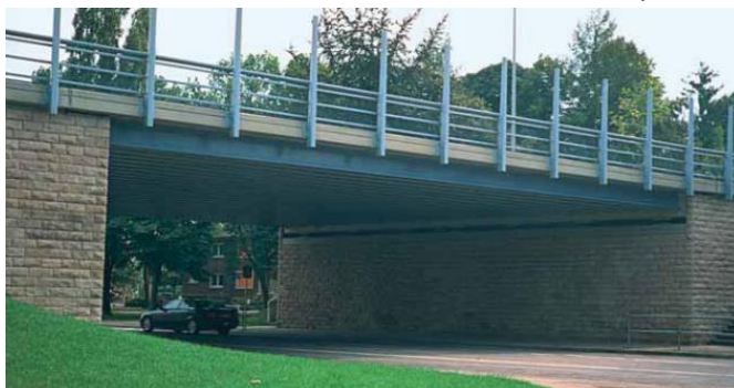
Figure 129 Example of a 19m-span composite steel bridge
