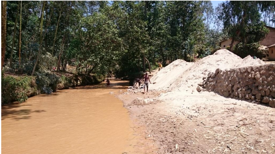
Figure 66: Sebeya (looking upstream): water spills over the stone-made wall and floods
