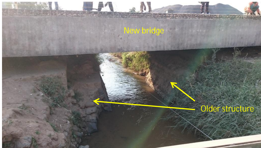
Figure 70: New bridge on river Pfunda (road to Rutsiro)
