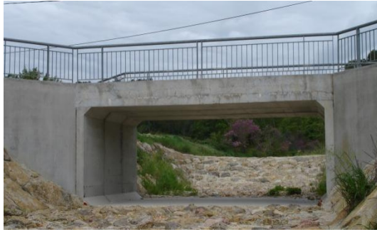
Figure 130: 5 x 2.5m culvert
